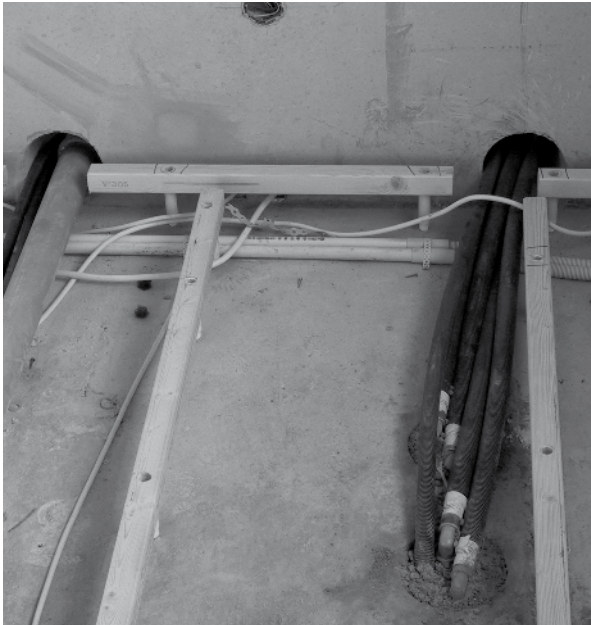
The services have been installed, ready to install the Nivell floor.
